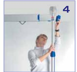
Fix the end cap to lock the rail in place.
